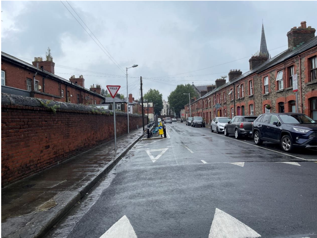
This zig-zag/(chicane) on Longwood Avenue, Portobello is created by having parking on alternating sides of the street. This can be done with parallel or other parking layouts.
