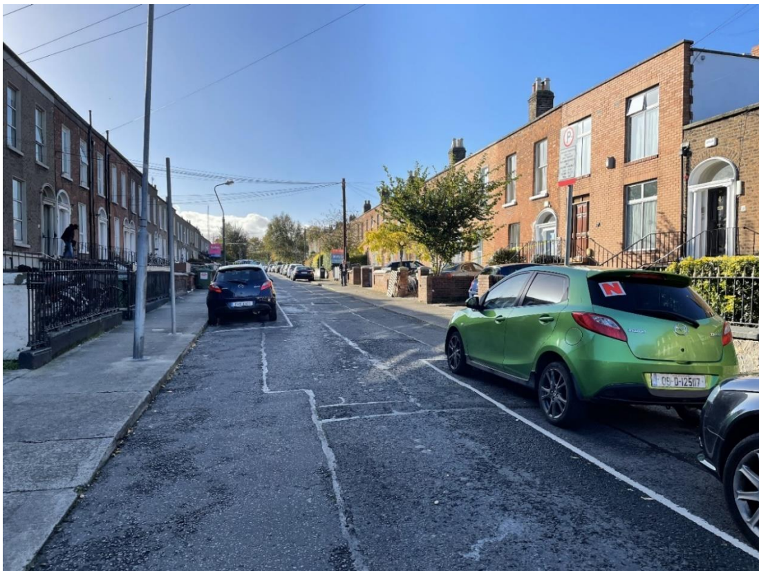
This zig-zag/(chicane) on Longwood Avenue, Portobello is created by having parking on alternating sides of the street. This can be done with parallel or other parking layouts.
